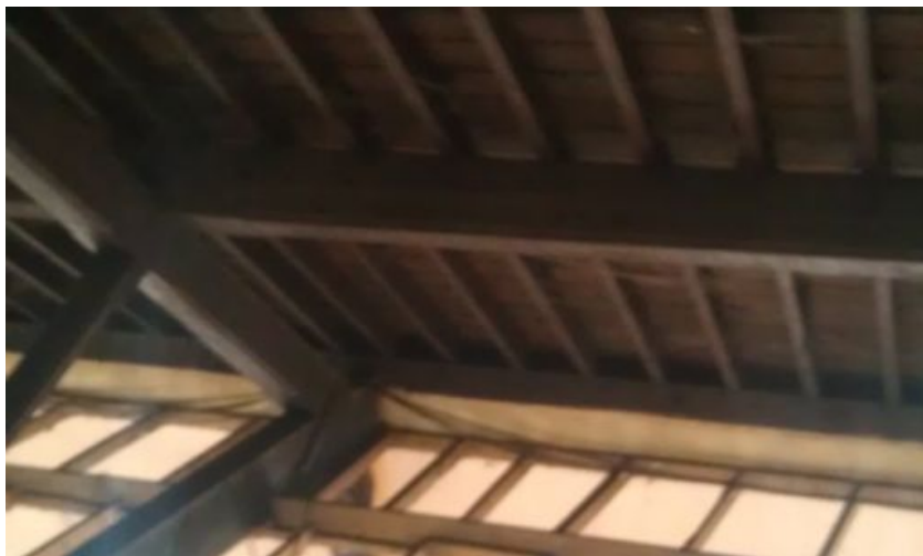
fig 6.21, Interior view of roof ceiling
