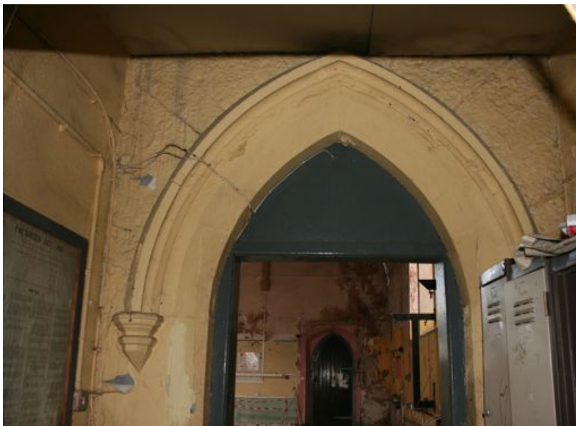
fig 6.15, Exterior of South Doorway (note door is missing)
