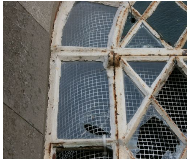
fig 6.8, Detail of Glazing
