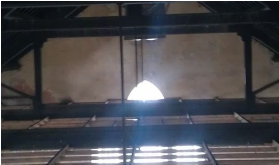
fig 6.17, Roof Space looking east
