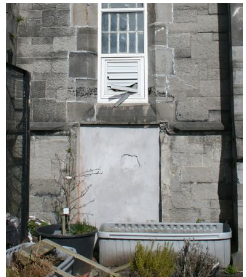
fig 6.10, Window with modern blockwork panel to base
