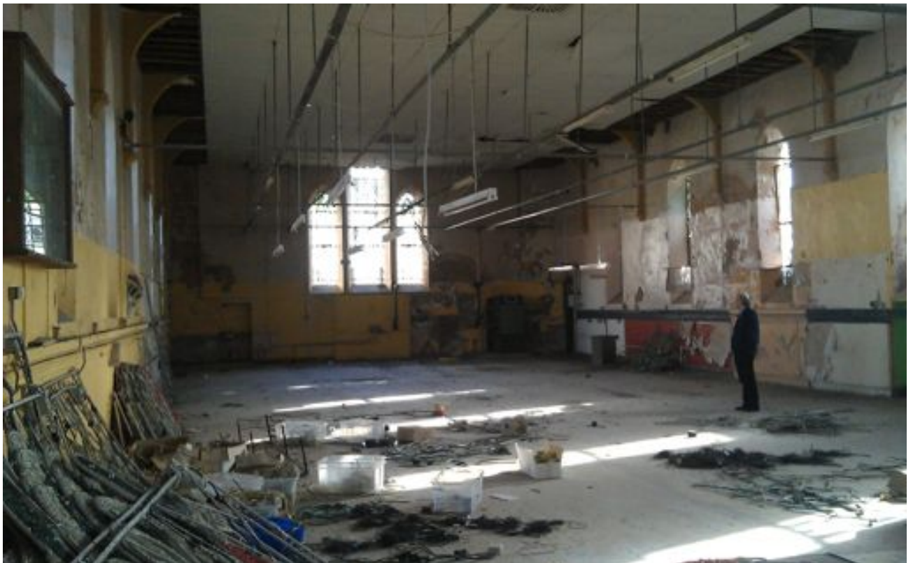
fig 6.12, Interior of church - looking east
