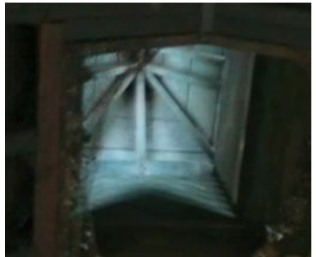
fig 6.20, Interior view of roof vent
