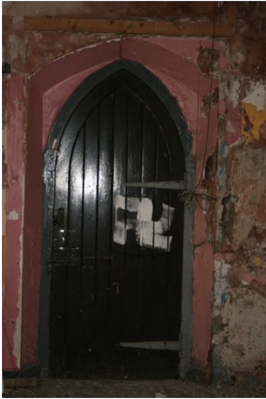
fig 6.13, North Entrance Door
