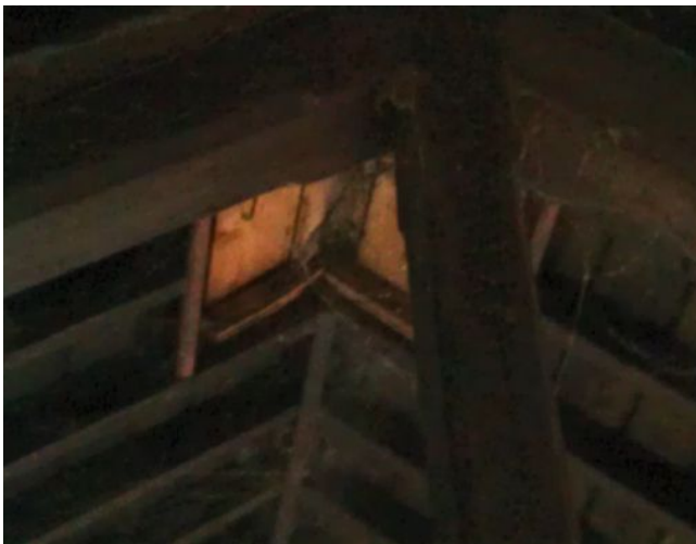
fig 6.19, Trimmed out rafters for vents that have been removed
