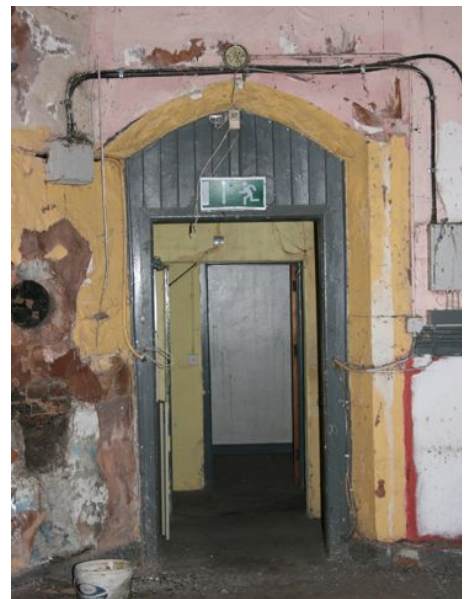
fig 6.15, Interior of South Doorway
