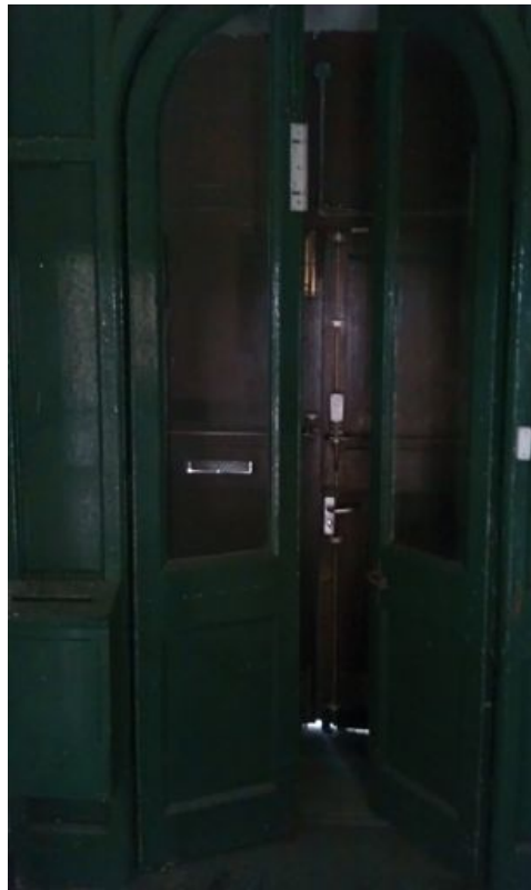
fig 6.14, Existing internal door
